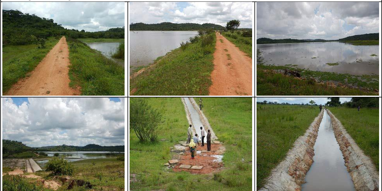
02. Ulyanyama Dam Irrigation Scheme, Sikonge District, Tabora Zone
